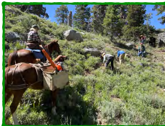
Building a bypass trail.
